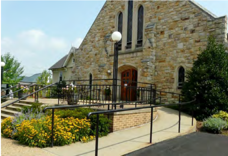
The ramped entrance and piazza provide access to worship and fellowship at the 2010 Open Hearts Award winning St. Patrick Catholic Church in Lexington, Virginia.
